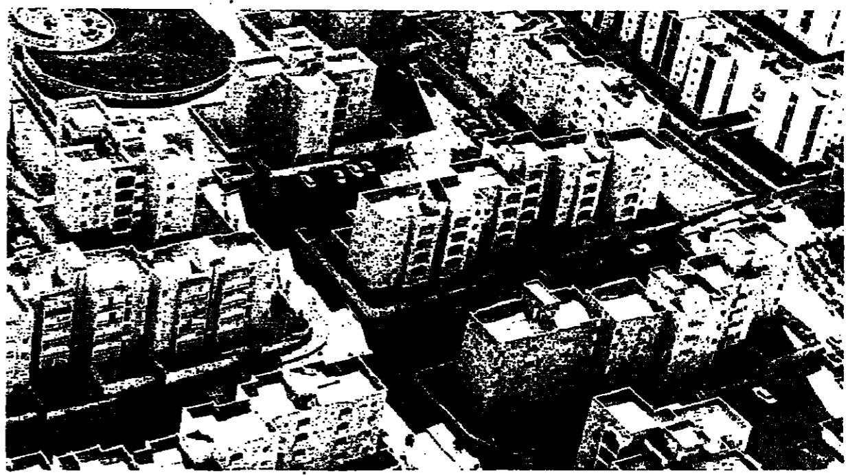
Ramat Eshkol — over-built residential structures, says James Kravitz.
